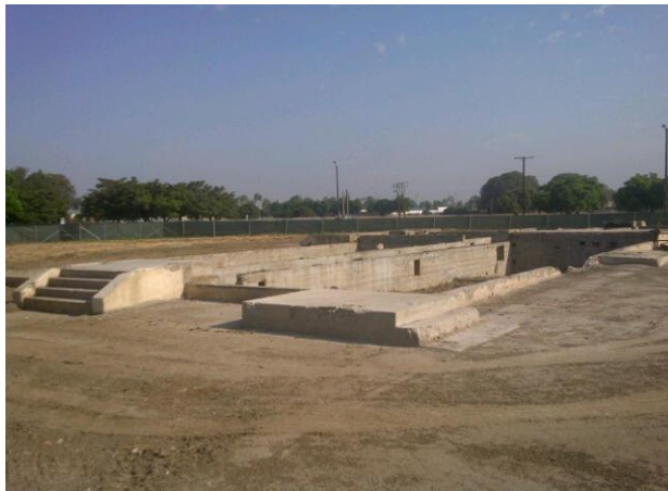
Bldg 4 – Slab Condition
