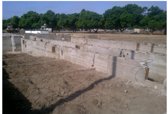
Bldg 4 – Sub-surface Foundation Condition
