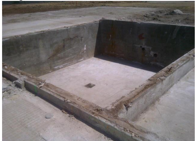
Bldg 300 – Basement Condition ready for backfill
