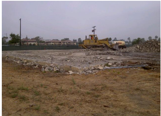
Bldg 166 – Slab Condition
