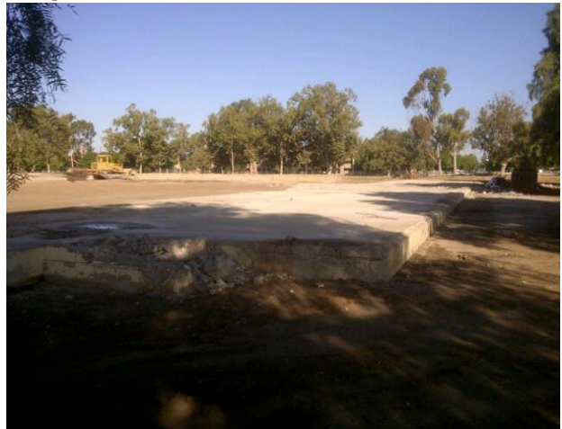
Building 134 – Slab Condition
