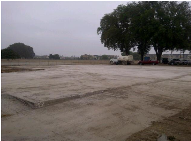
Bldg 165 – Slab Condition
