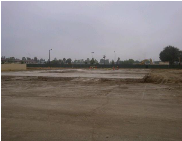
Bldg. 300 – Slab Condition
